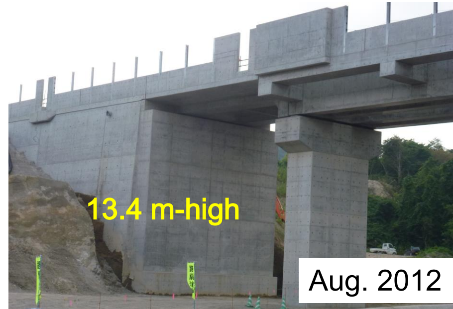
GRS Bridge Abutment at Mantaro for Hokkaido Shinkansen
