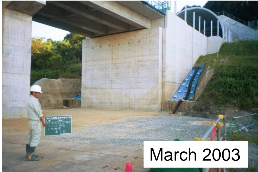
First GRS Bridge Abutment at Takada for Kyushu Shinkansen
