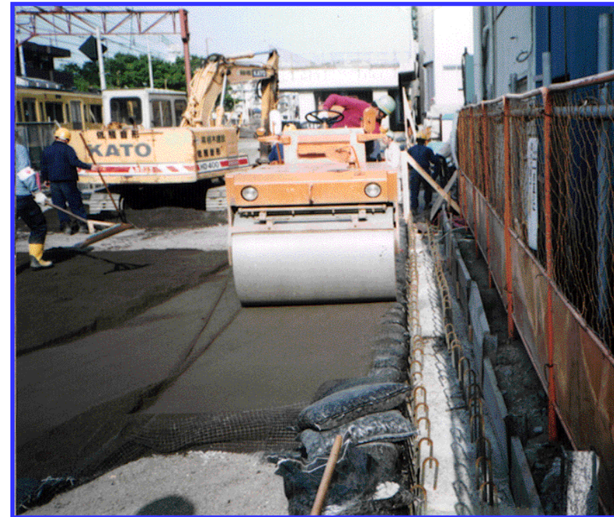
2) Placing geosynthetic & gravel bags
