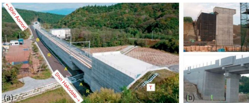
Figure 23.8 (a) A view of a variety of GRS structures at the Mantaro section of the south part of the Hokkaido Shinkansen and (b) GRS bridge abutment (13.4-m high) during and after construction near tunnel.
